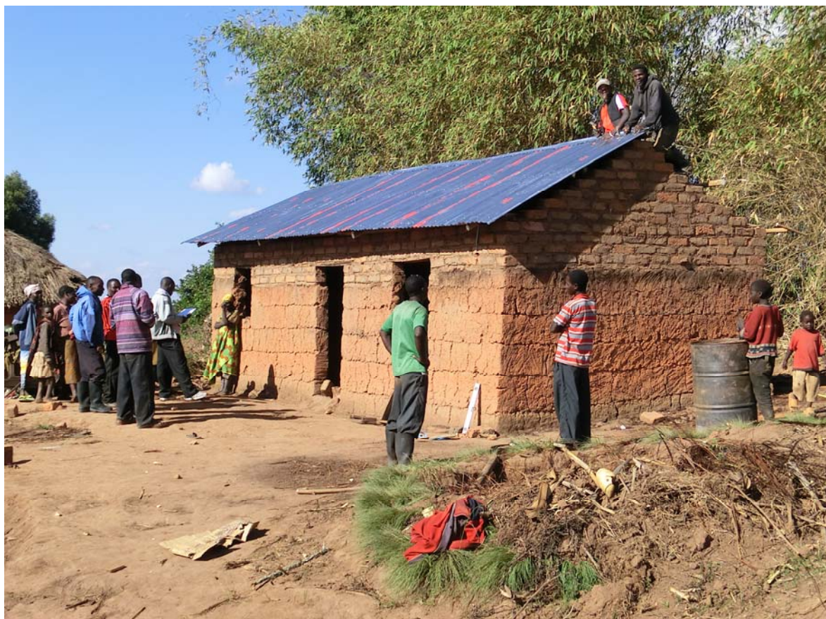
House with well-preserved clay ramped walls, which was increased with Sun-dried mud bricks and covered with corrugated iron. Left in the picture - the Committee visited the construction progress and registers the need for doors and windows. Right viewing craftsmen in roofing work.
