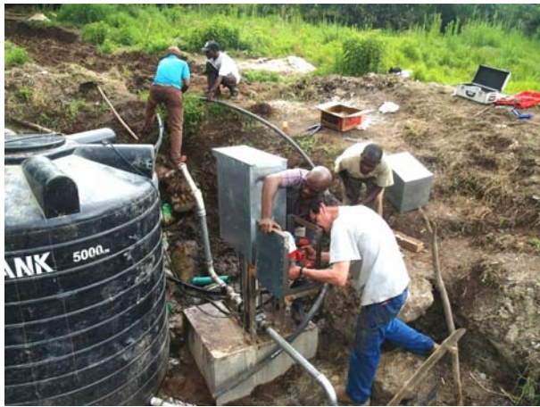
Installation of electric water pump at the spring tapping of VTC Ibwanzi.
