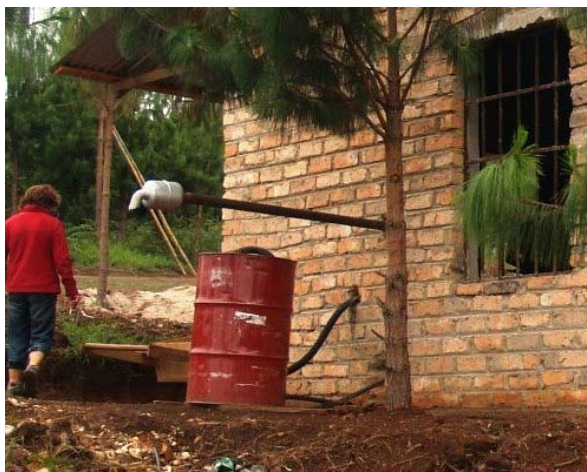
Exhaust and cooling drum for the generator in the PH.
