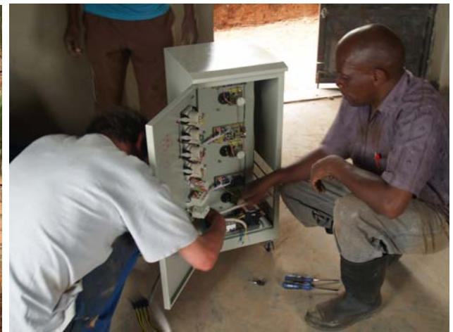
Connection of rectifier
