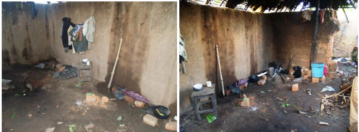
In the old house: apertured roof, damp walls and damp soil, the clothes will not dry, hopelessness and lethargy may spread
