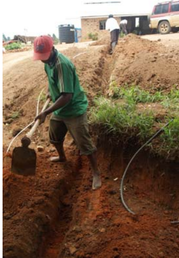
Electrical cable is routed from the Powerhouse to VTC building
