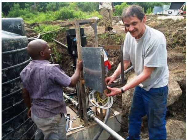
Installation of electric water pump at the spring tapping of VTC Ibwanzi.
