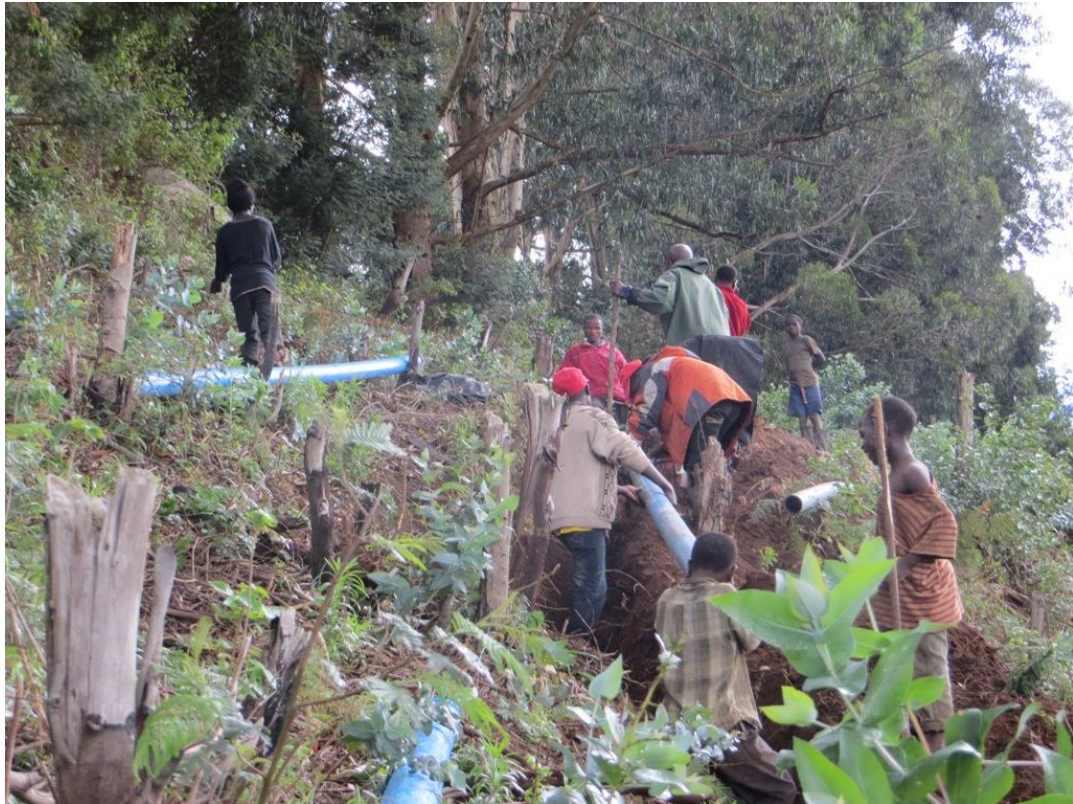
Fig Pipelaying on the ground - the picture below: In the valley floor, the stronger pipes must be welded
