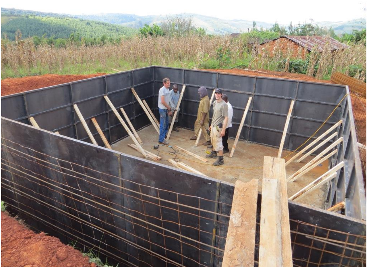
Fig. A reusable steel formwork for the construction of all water tank was produced in the RDO – Metal Workshop
